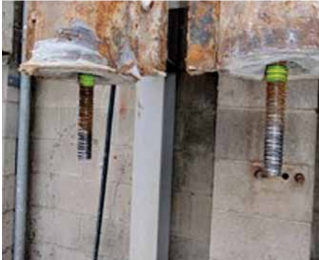
R27 de-bonded secura bolt before applying load
