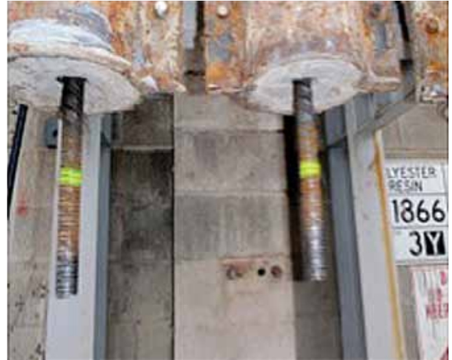
R27 de-bonded secura bolt after load has been applied
